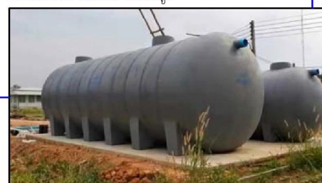
Water tank underground finished ບ່ອນເກັບນໍ້າແບບສໍາເລັດຮູບ
